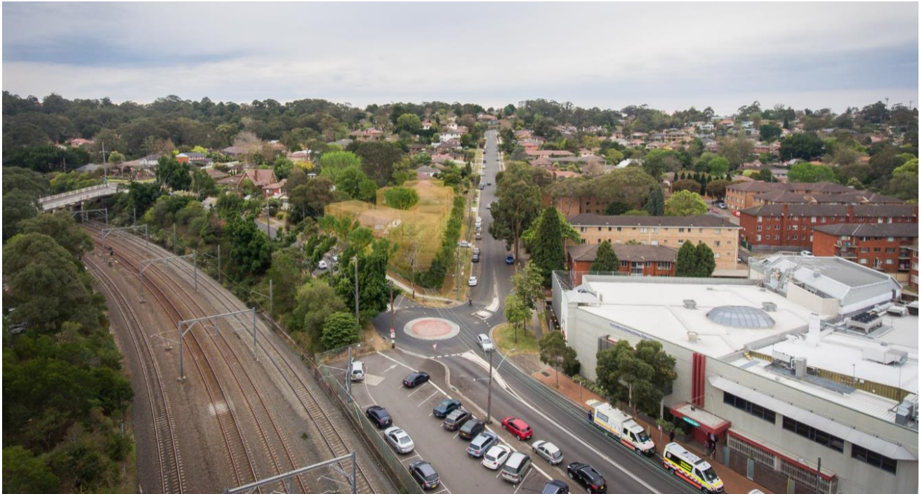
Figure 12 – Envelope Massing from above the corner of Ryedale and Terry Roads
